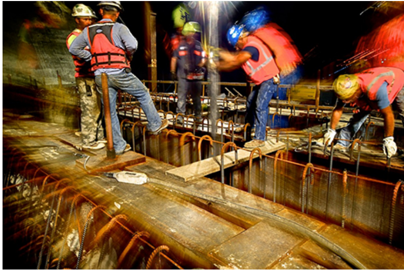
1st: Nick Roberts Placing the Concrete for Pier Four
