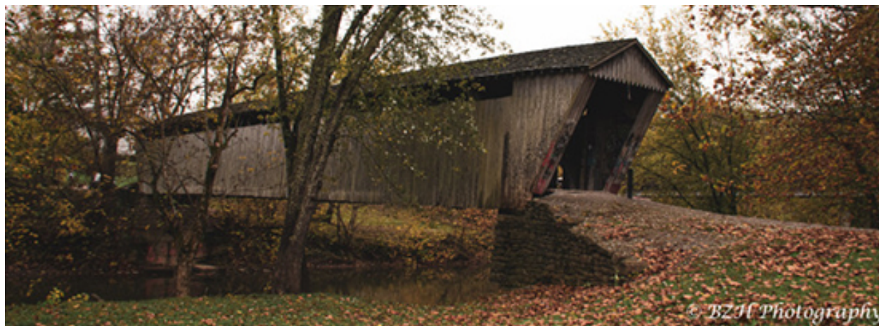
Switzer Covered Bridge
