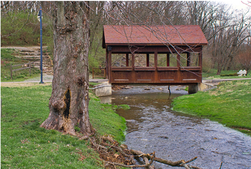
Walking Bridge in Greenway Park
